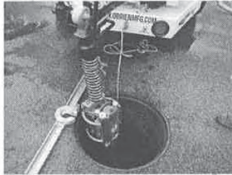
Environmental Services inspects its stormwater pipes using a hydraulic-powered video camera
