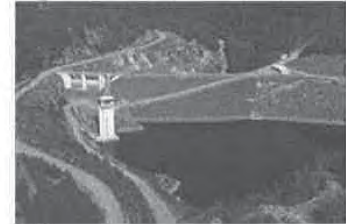
Howard Hanson Dam
