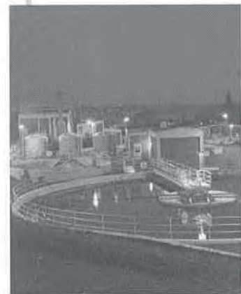
North End Wastewater Treatment Plant
