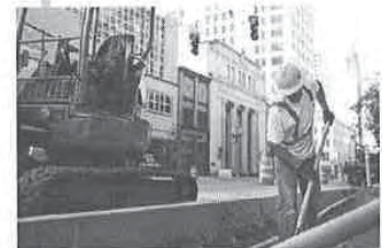
Construction on Pacific Ave
